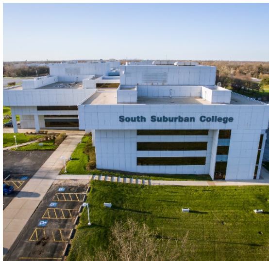
The South Suburban College Main Campus in South Holland, Illinois.
